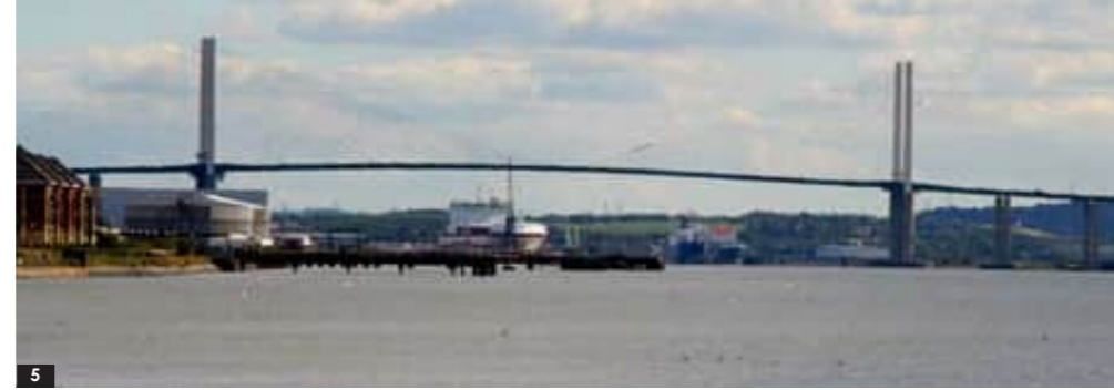
Fig. 5 The Queen Elizabeth II Bridge joining the M25 as it crosses the River Thames seen from Rainham Marshes
